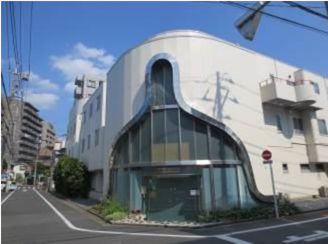
< 外観 External appearance >
