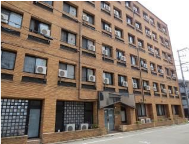
< 外観 External appearance >
