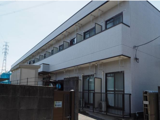
< 外観 External appearance >
