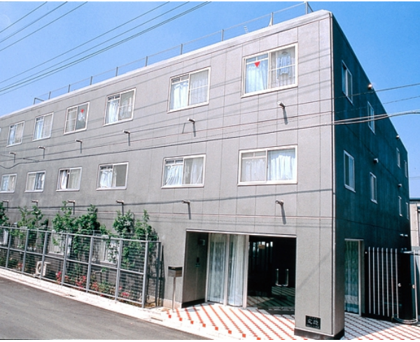
< 外観 External Appearance >
