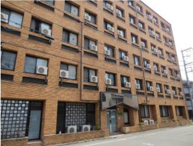
< 外観 External Appearance >
