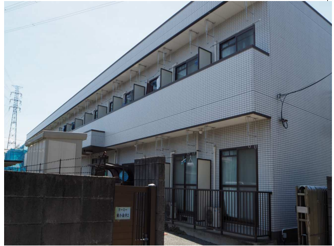
< 外観 External Appearance >
