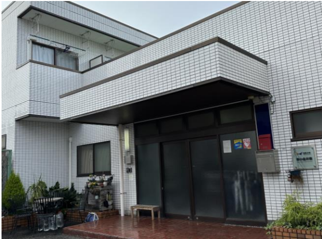
< 外観 External appearance >
