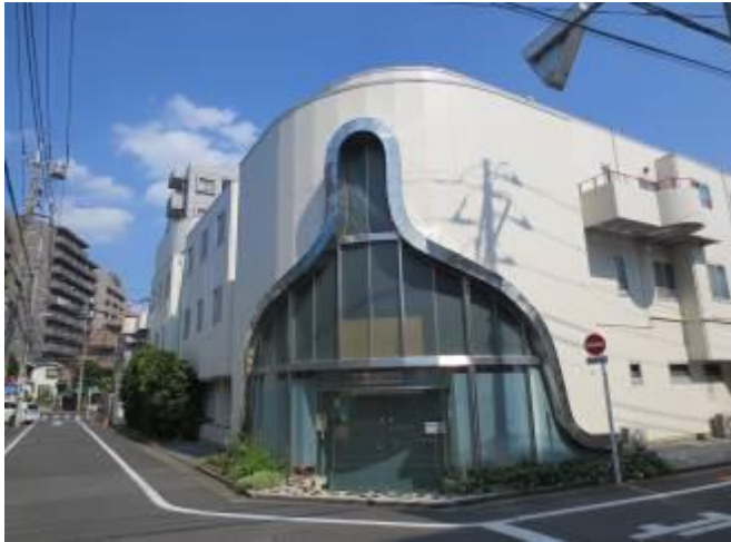
< 外観 External appearance >
