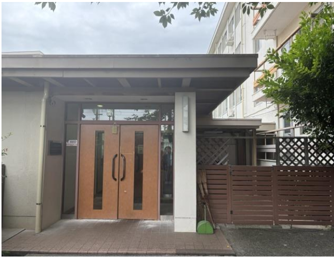
< 外観 External appearance >
