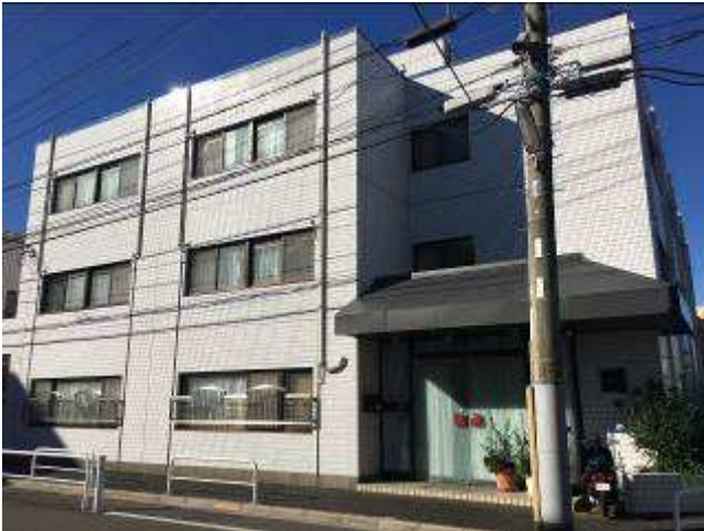
< 外観 External Appearance >
